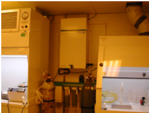
Fig 2. The E-pure water purification unit. It is hanging on the wall between the two fume hoods.
