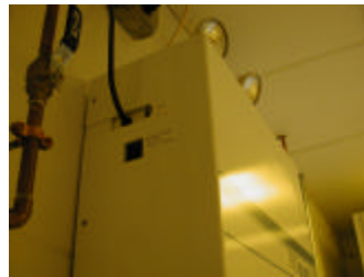
Fig 5. The shutoff valve is on the left side of LP. The 'power' button is on the left sidewall of LP.
