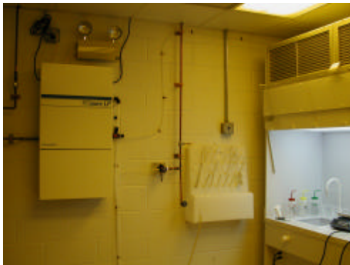
Fig 1. The Barnstead ROpure LP reverse osmosis system. It is hanging on the center of the left wall from the entrance.
